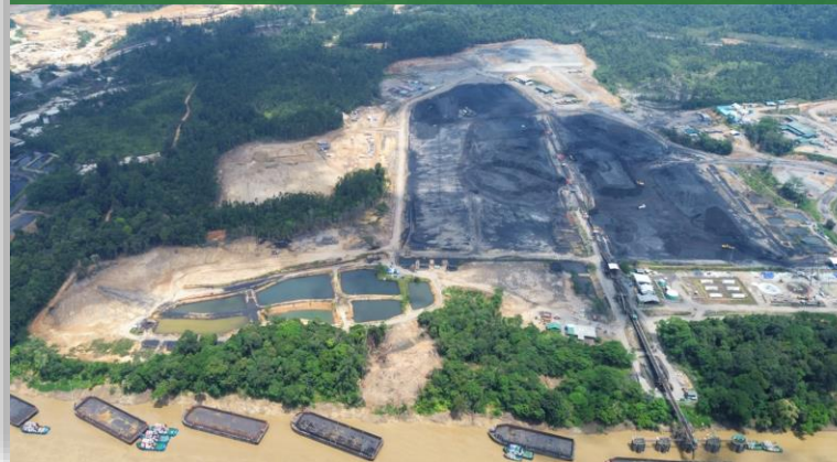
Barge loading conveyor area
