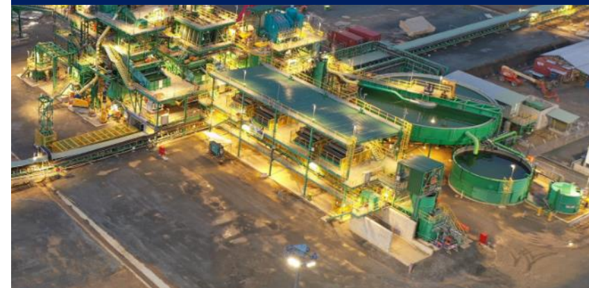
Washing Plant : 525 tph (max: 550 tph)
