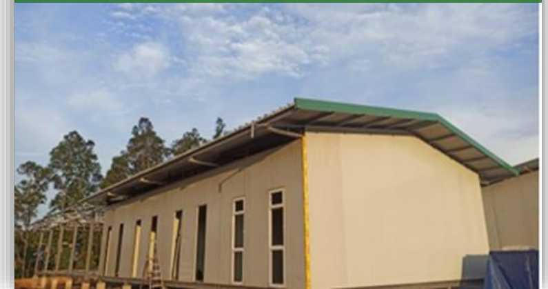
Employee dorms' construction
