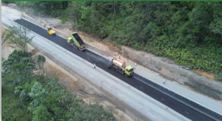
Hauling road progress
