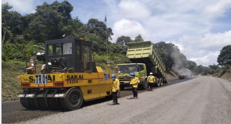
Hauling Road Upgrade
