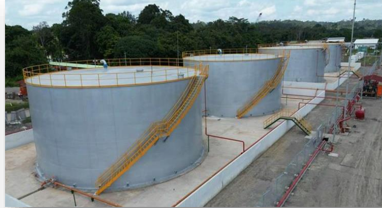
Fuel Storage Tank
